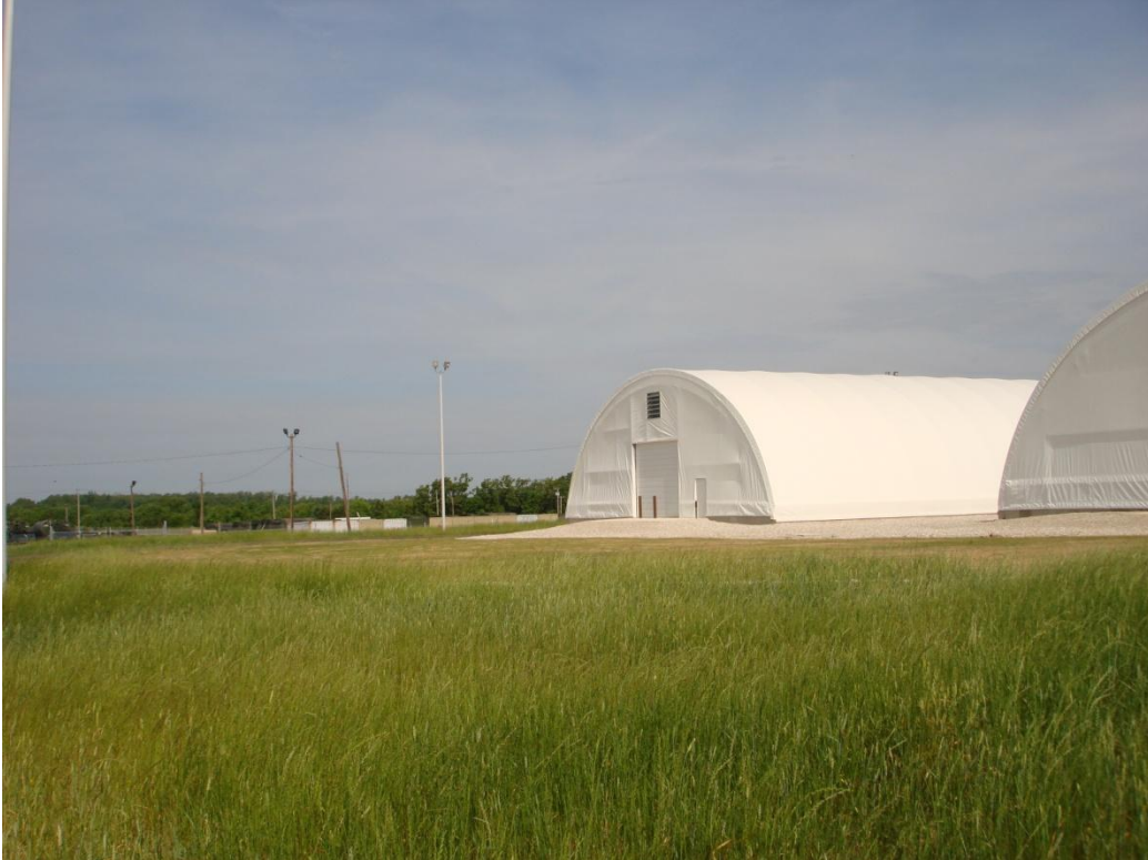
Facing Northwest towards open area and temporary structures
